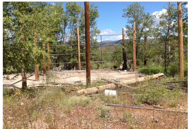
PHOTOGRAPH No. 25 View of former logger shop
