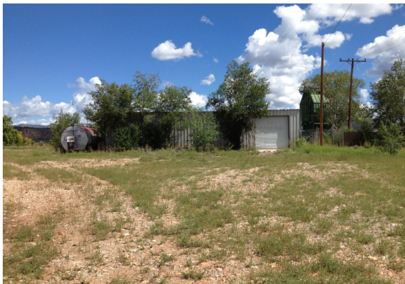
PHOTOGRAPH NO. 19 View of fuel pump and tank facing east
