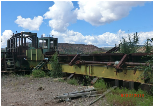
PHOTOGRAPH NO. 15 View of saw mill equipment looking northeast
