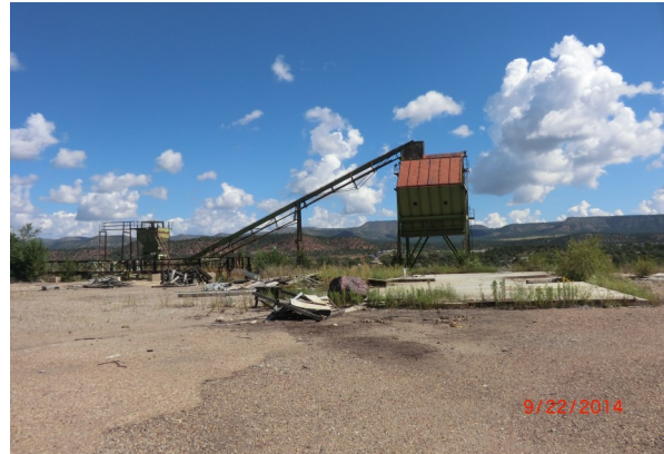
PHOTOGRAPH NO. 2 View of wood chipper and concrete pad looking east
