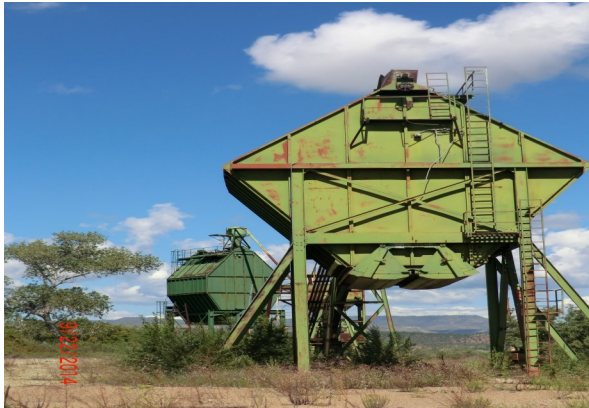
PHOTOGRAPH NO. 5 View of front of wood chipper looking north
