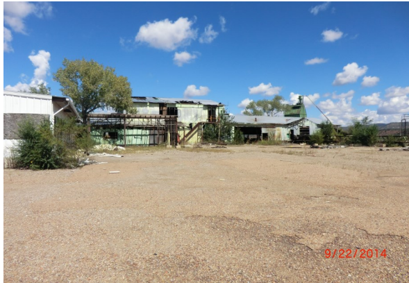
PHOTOGRAPH NO. 1 View of the saw mill looking north
