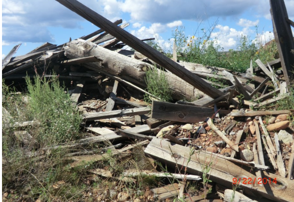
PHOTOGRAPH No. 38 View of debris pile looking west
