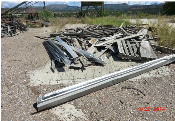
PHOTOGRAPH No. 40 View of debris pile looking east
