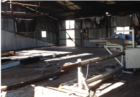
PHOTOGRAPH NO. 26 View of the inside break room structure
