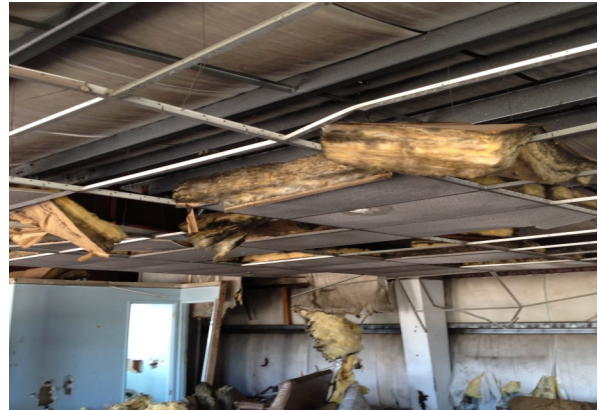
PHOTOGRAPH NO. 27 View of ceiling in break room structure
