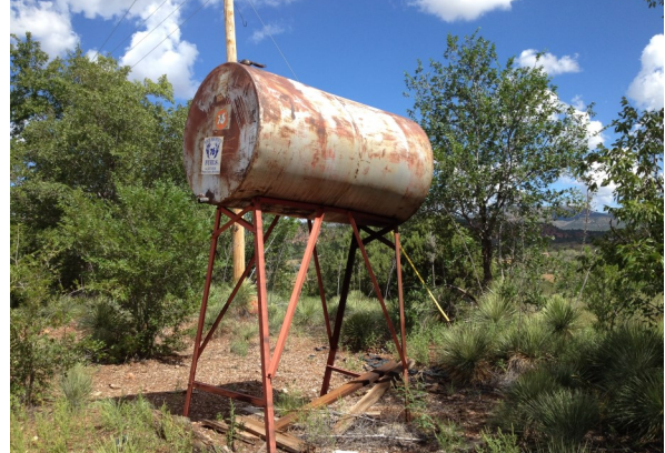
PHOTOGRAPH No. 23 View of tank looking northeast
