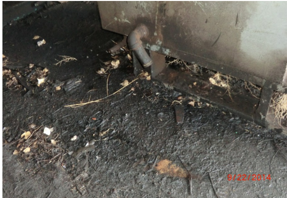
PHOTOGRAPH NO. 13 View of inside saw mill at hydraulic fluid
